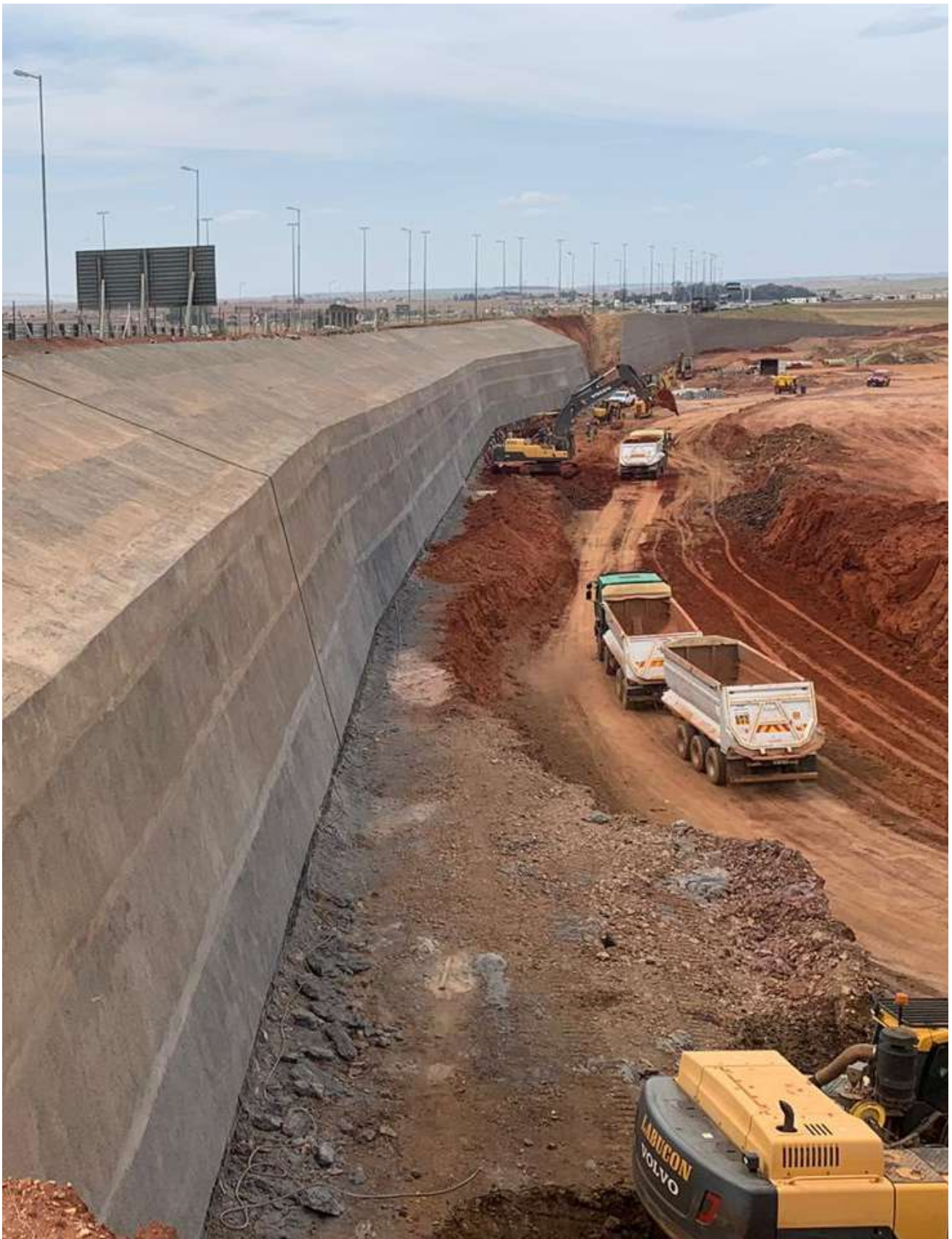
RAILWAY EMBARKMENT SLOPE STABILISATION
