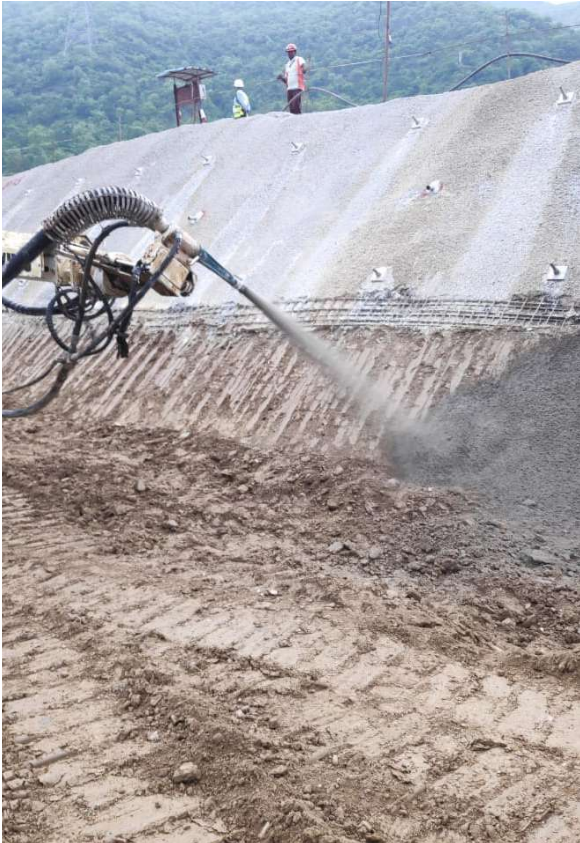
MECHANICAL SHOTCRETE SPRAYING FOR SLOPE STABILISATION
