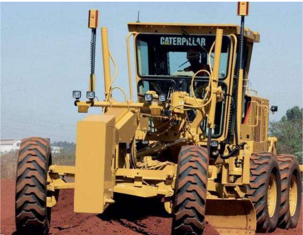
SITE CLEARING AND GRADING
