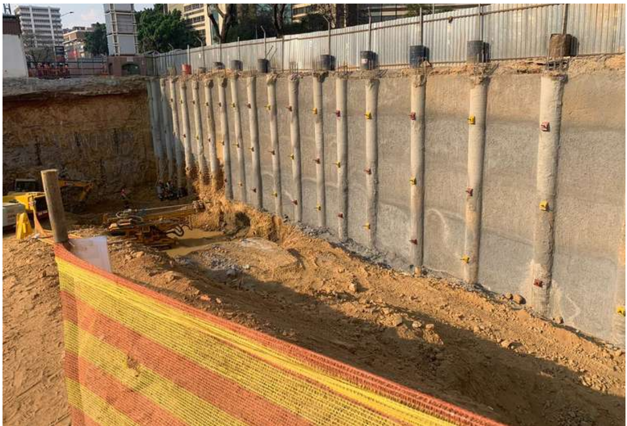
DEEP BASEMENT SUPPORT WORK
