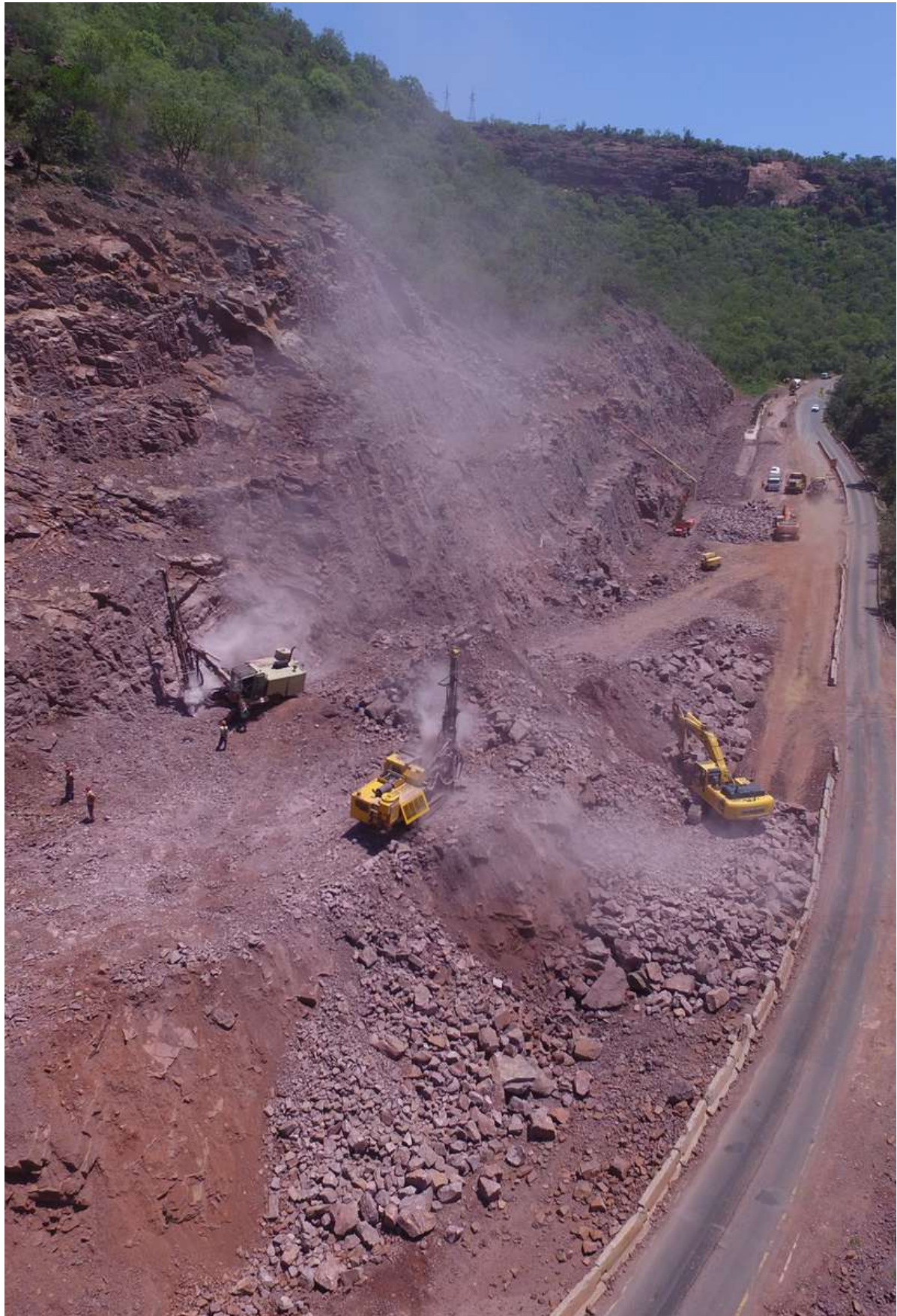
ESCARPMENT CUTTING WITH A DRILL & BLAST METHOD AND HIGH WALL SUPPORT
