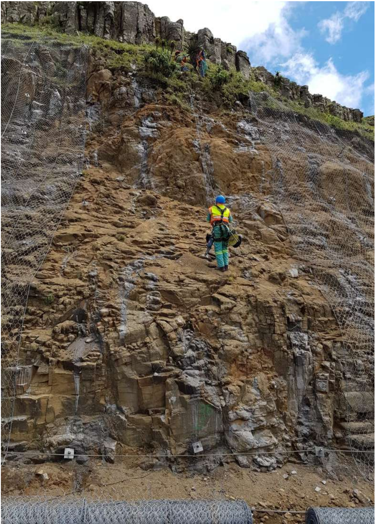
SLOPE STABILISATION USING MESH
